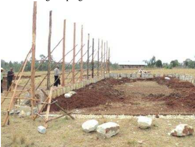
Pict 7: FTC under construction, Enmore, March 2011
