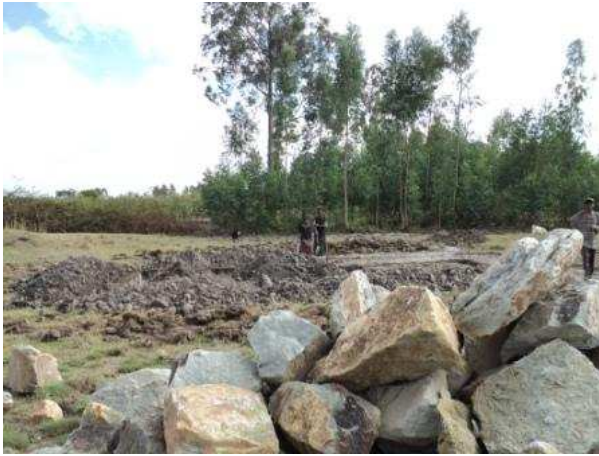
Pict 5: Construction site of veterinary health post
