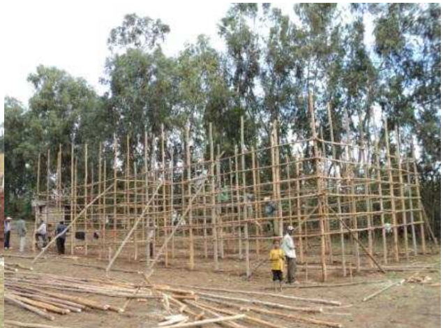
Pict 8: FTC under construction, Mirab-Badewacho, March 2011
