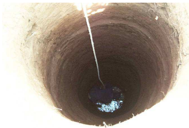
Pict 2: Hand dug wells' inside view during construction
