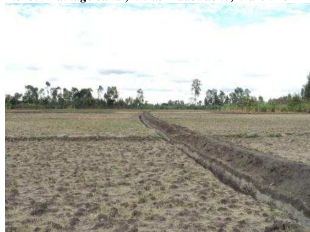
Pict 3: Drainage canal, Mirab-Badewacho, March 2011
