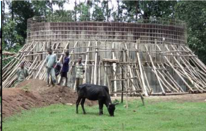
2. Belete spring reservoir construction
