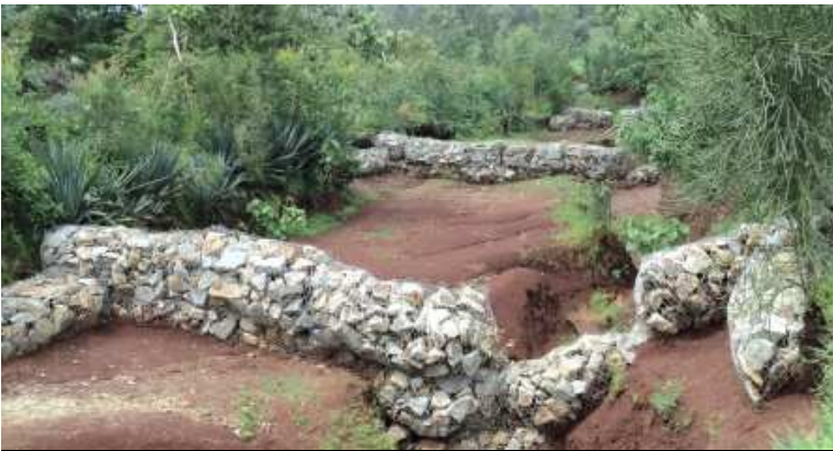
6. Mirab-Badewacho – Gabion check dams (still without other plantations)
