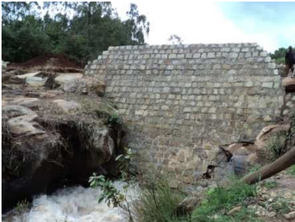
1. Derkeye river diversion weir – dam construction
